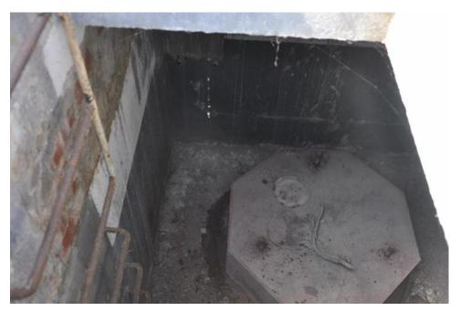
Figure 28. BES B'5 (#5) Interior with Octagonal Concrete Pad for DPF. Source: Page & Turnbull, 2014.
