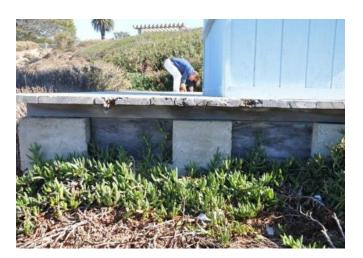
Figure 60. Detail of Radio Direction Finder Building Remaining Foundation (#13). Source: Page & Turnbull, 2013
