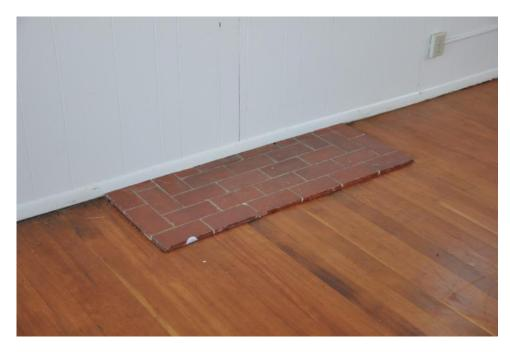
Figure 41. U.S. Navy Radio Station & Barracks (#6), a brick hearth remains where the chimney was demolished. Source: Page & Turnbull, 2013
