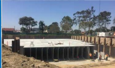
Pre-Cast Subsurface Infiltration Facility
